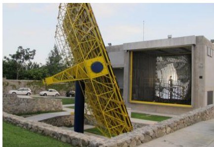
Figure 1. High Radiative Flux Solar Furnace at CIE-UNAM.
